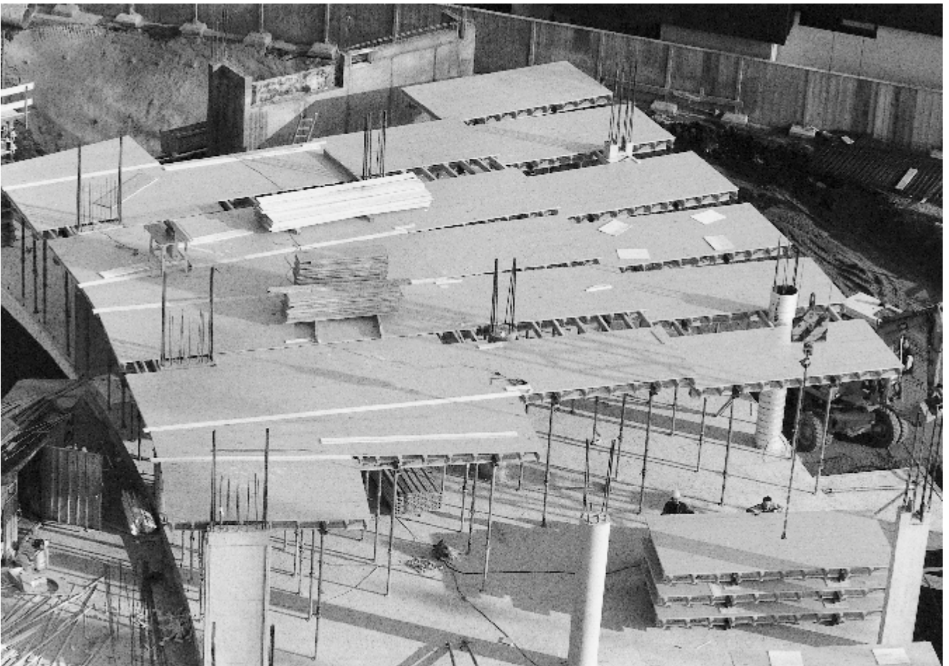
Site: "Chirurgie West" hospital extension, Salzburg
