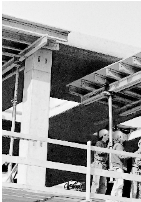
Site: Warehouse for Messrs. Klotzner, Linz, Austria
