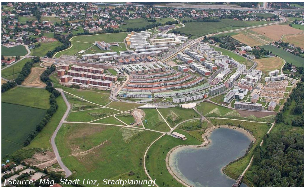
195. ábra solarCity Linz-Pichling
