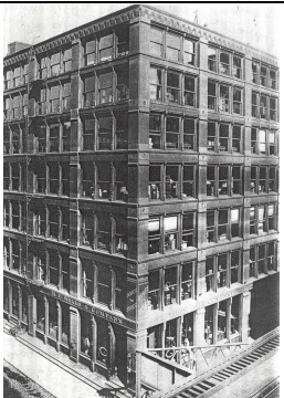
Jenney: Leiter Building 1879
