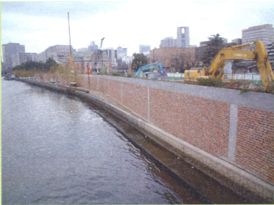
Decoration With a Brick For the Temp. Revetment
