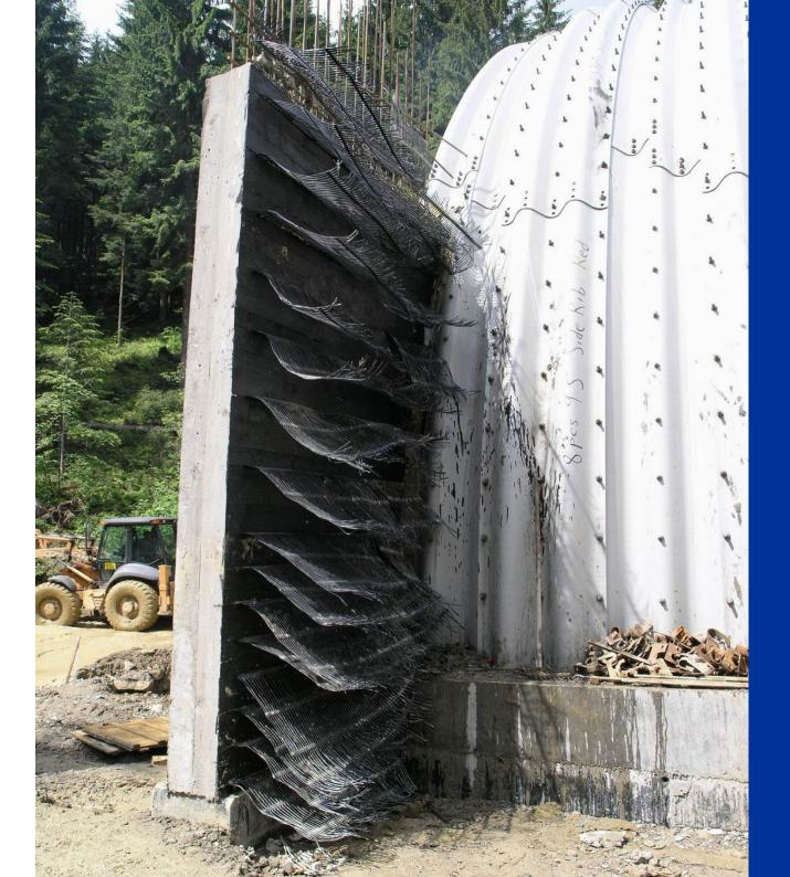
Joining of concrete panel to steel arch
