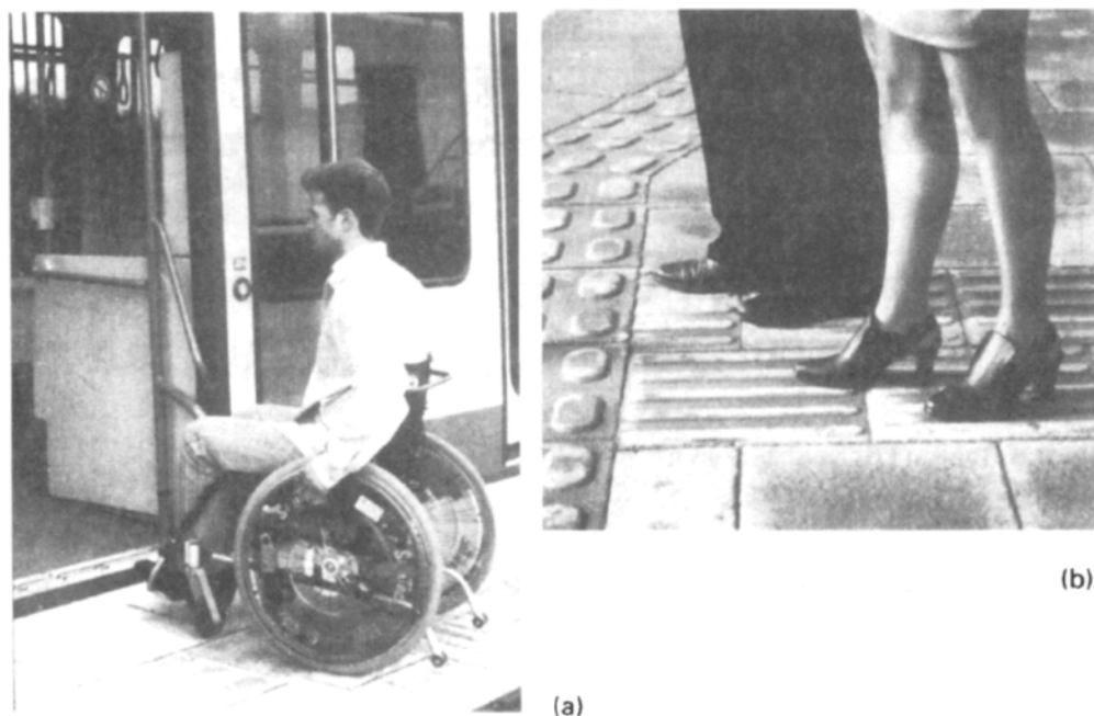
Fig. 9.7 (a) Floor level vehicle access, with (b) tactile paving defining the platform edge and door position 20
