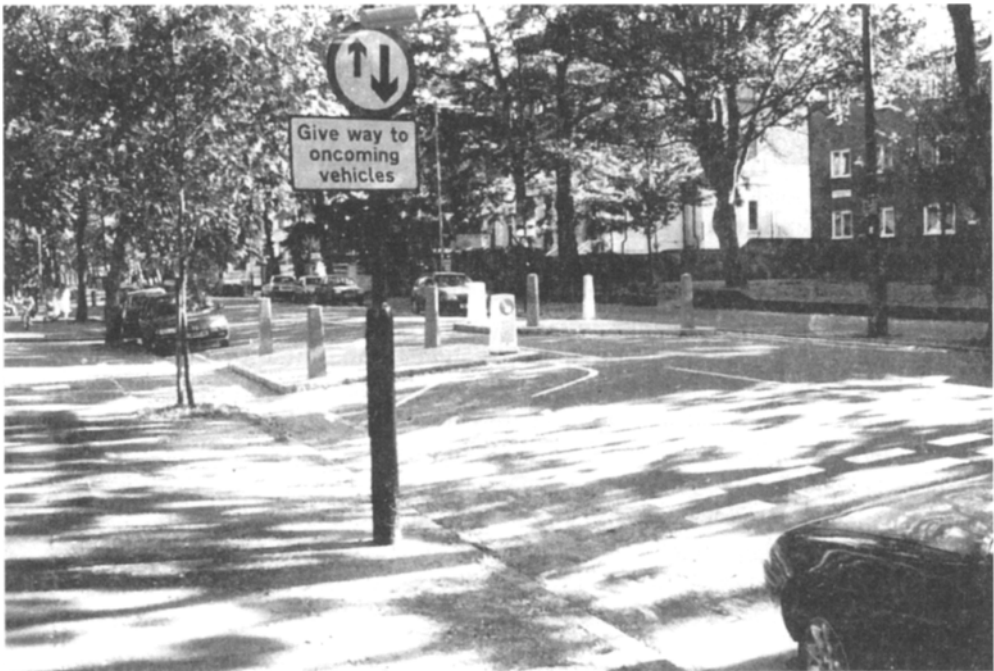
Fig. 25.2 Chicane in a residential street
