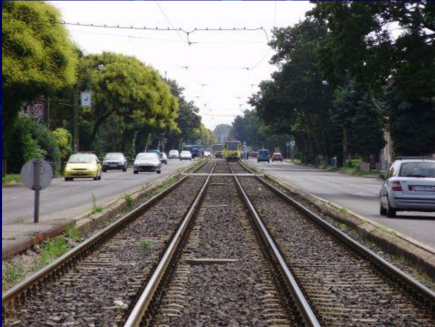
Separated tram line (Miskolc)
