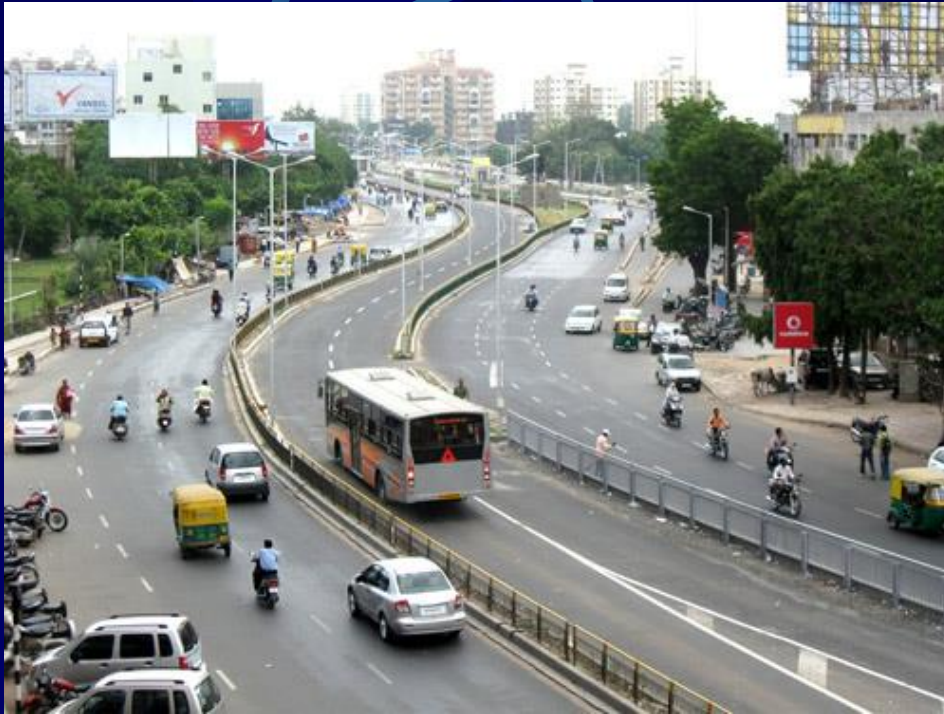
Separated bus corridor (India)
