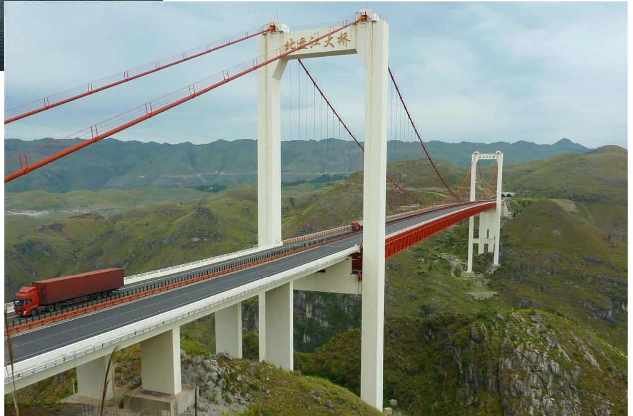
Beipan River Hukun Expressway Bridge
