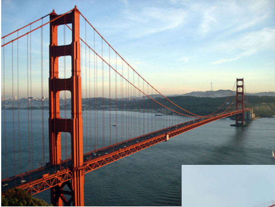
Golden Gate bridge, CA
