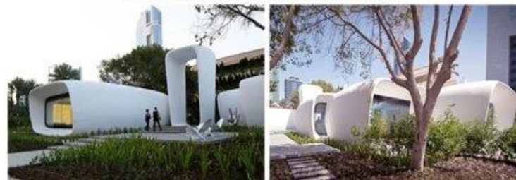
Media office buildings (Dubai)
