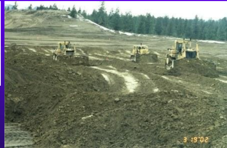
Bulldozers at work: embankment fill
