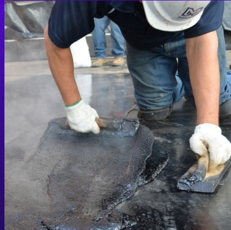
Mastic Asphalt cooker and using its product for bridge repair
