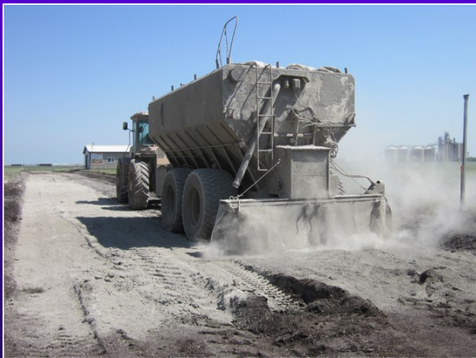
Cement stabilization of granular soil subgrade Timár 2019
