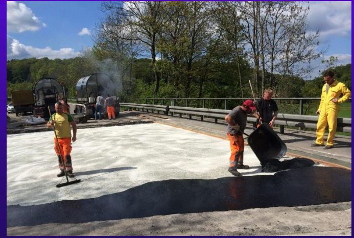
Mastic Asphalt cooker and using its product for bridge repair
