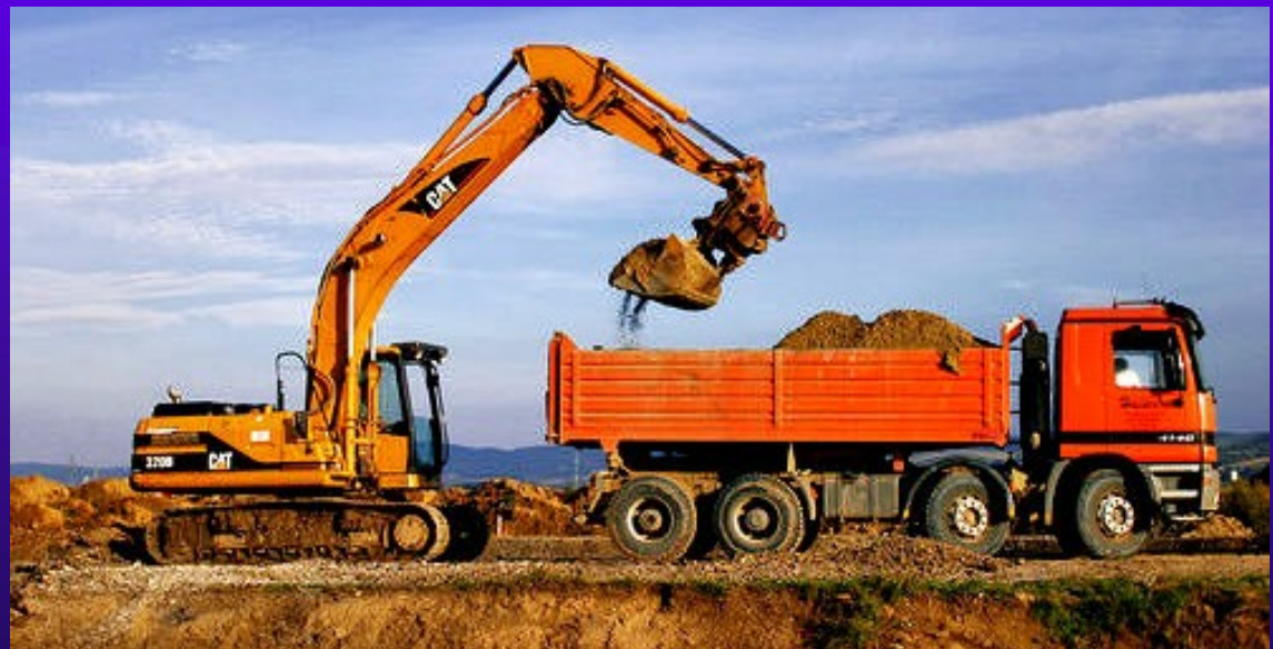
Excavating soil from cut area or borrow pits and moving it to fill area by dump trucks
