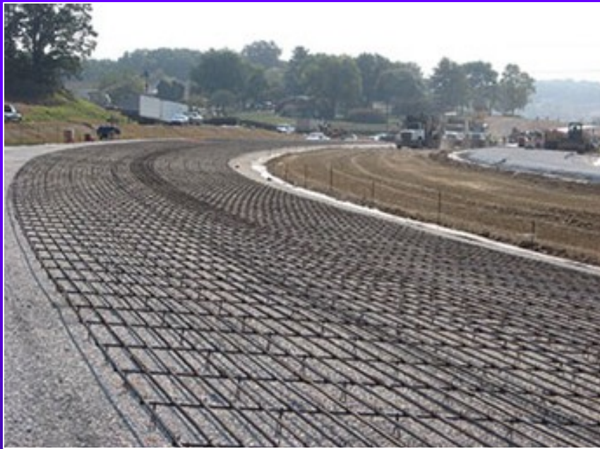
Continuous reinforcement assemblies with steel rebars
