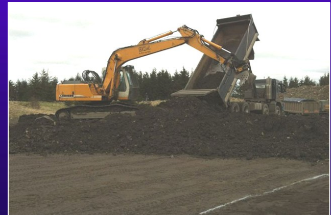
Excess soil disposal area
