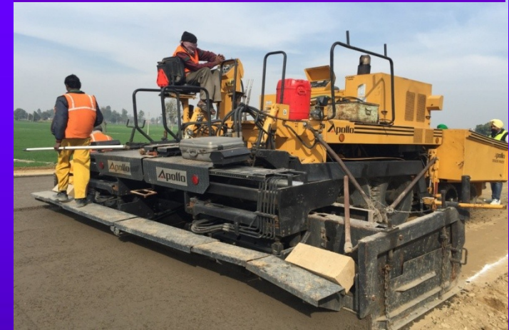
Laying of dry lean concrete (DLC)
