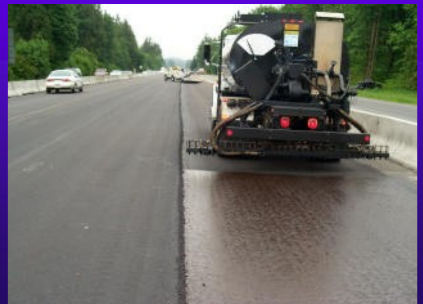
Good tack coat coverage
