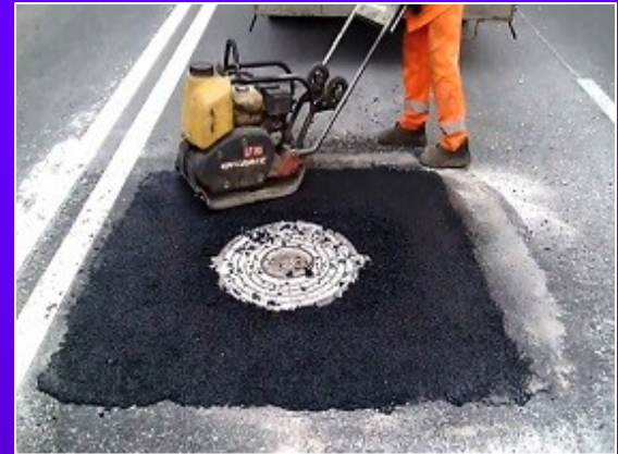
Cold Mix Asphalt used for patching and levelling a manhole cover
