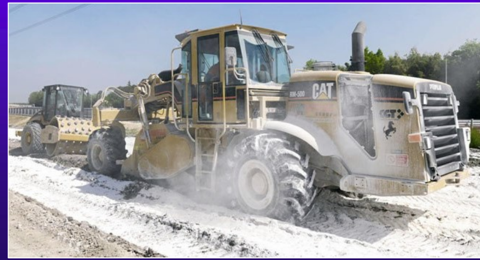
Using lime and fly ash as soil (clay, silt) stabilizers
