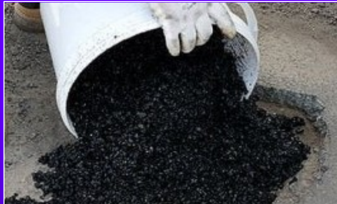
Cold Mix Asphalt used for patching and levelling a manhole cover
