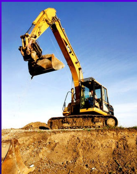
Excavating soil from cut area or borrow pits and moving it to fill area by dump trucks
