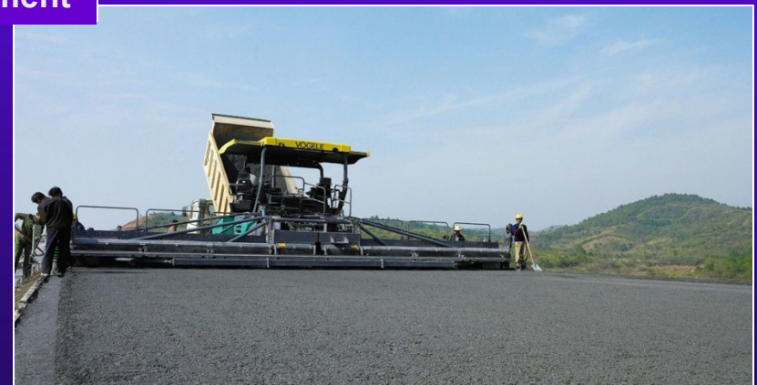
Placing a HMA base layer with a road paver
