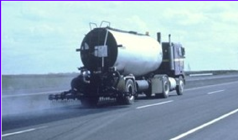
Spreading bitumen emulsion
