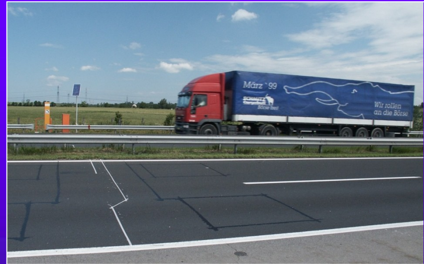
Typical layout of magnetic loops on the road surface
