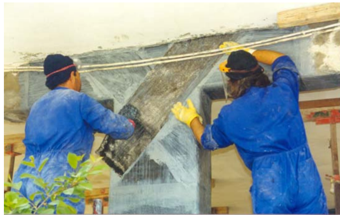
Fig. 1-2: Typical FRP applications as strengthening materials of RC structures: (a) flexural strengthening of slab; (b) flexural strengthening of beam; (c) shear strengthening and confinement of column; (d) wrapping of concrete tank; (e) shear strengthening of beam-column joint.
