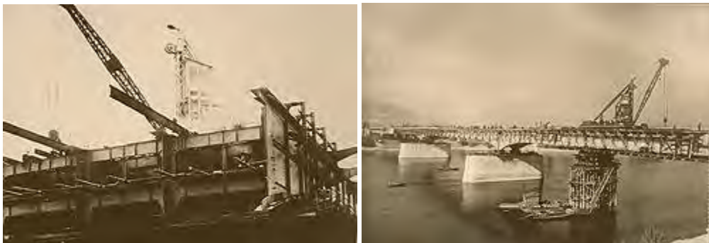
Figure 4.32 The erection of Árpád bridge.
