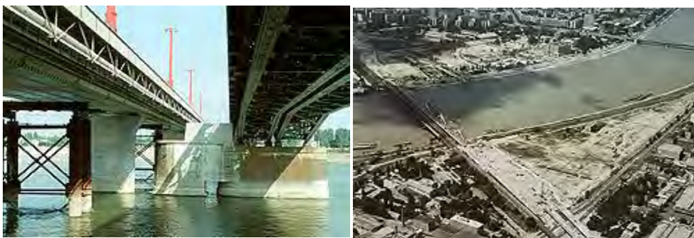
Figure 4.45 The general cross-section of the Southern Railway Bridge and the Lágymányos Bridges; the ensemble of the highway and railway bridges and aerial view of the bridge.
