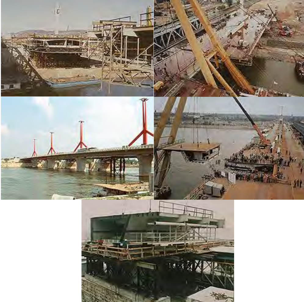
Figure 4.50 The erection of the bridge.
