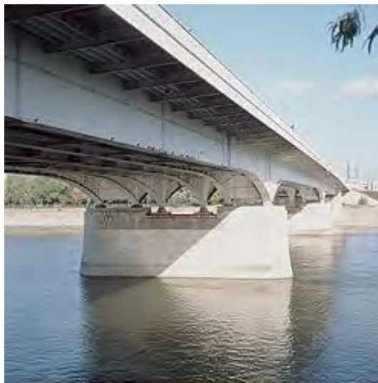
Figure 4.29 The Árpád bridge.
