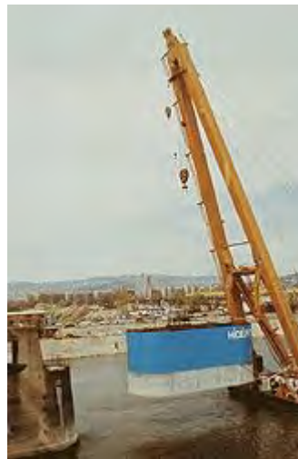
Figure 4.49 Lifting in of the upper casing element
