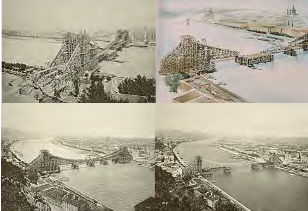
Figure 4.21 The erection of the bridge.
