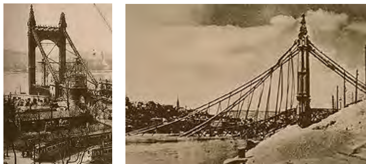
Figure 4.22 The bridge as blown up, 18 January 1945
