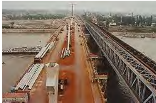
Figure 4.47 The erection of the columns
