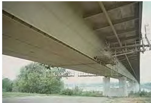
Figure 4.43 The piers of the bridge.
