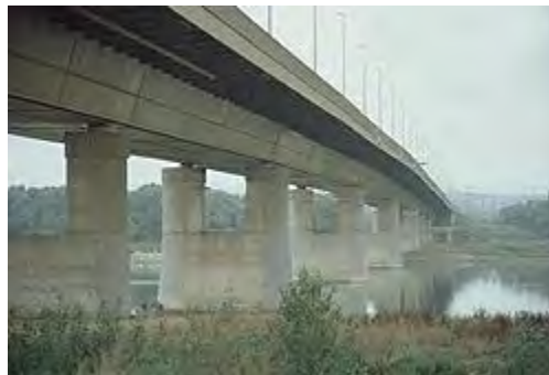
Figure 4.41 The piers of the bridge.
