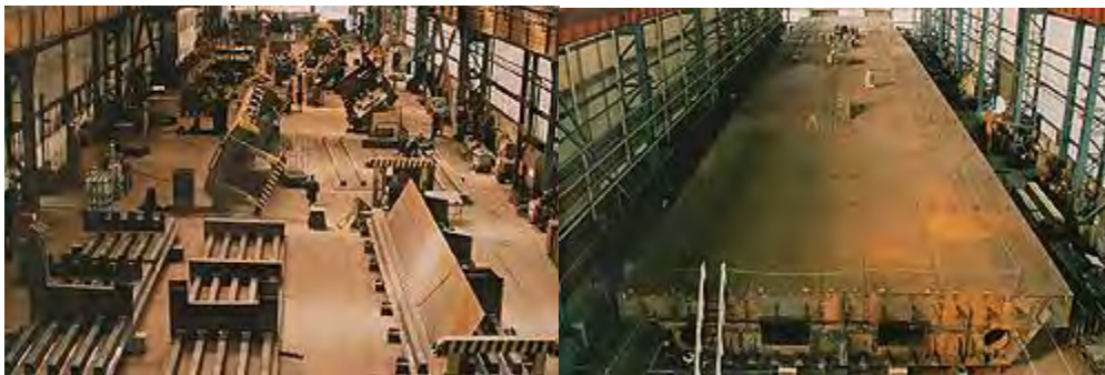
Figure 4.48 Laying of the elements of box girders and Pre-assembly of the main box girder sections at the GANZ-MÁVAG plant
