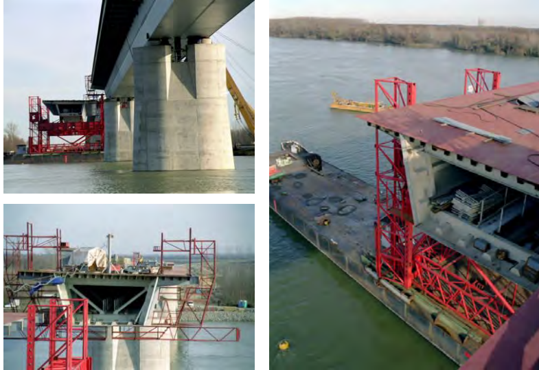
Figure 4.58 The erection of the bridge before lifting the last element.
