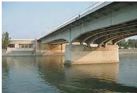
Figure 4.35 The three independent main beams, with two main girders each, are similar.
