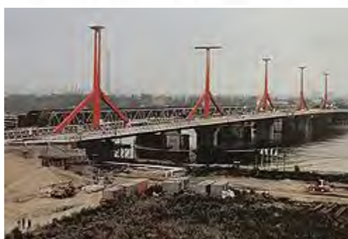
Figure 4.44 General view of the Lágymányos Bridge with the Southern Railway Bridge.
