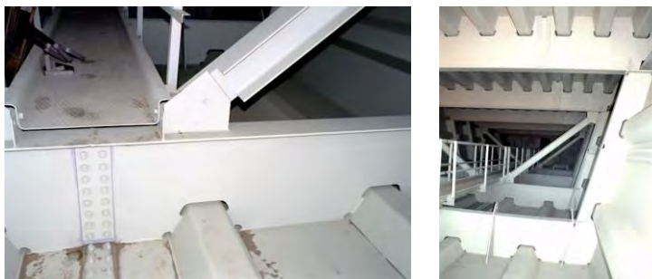
Figure 4.60 The lower flange plate and the cross bracing.
