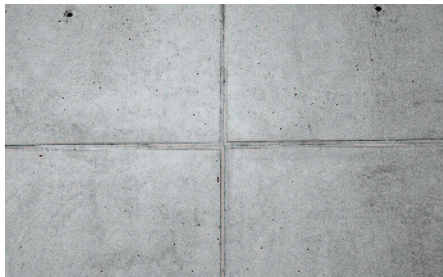
Keretlenyomat: B=18mm, T=1,5mm
